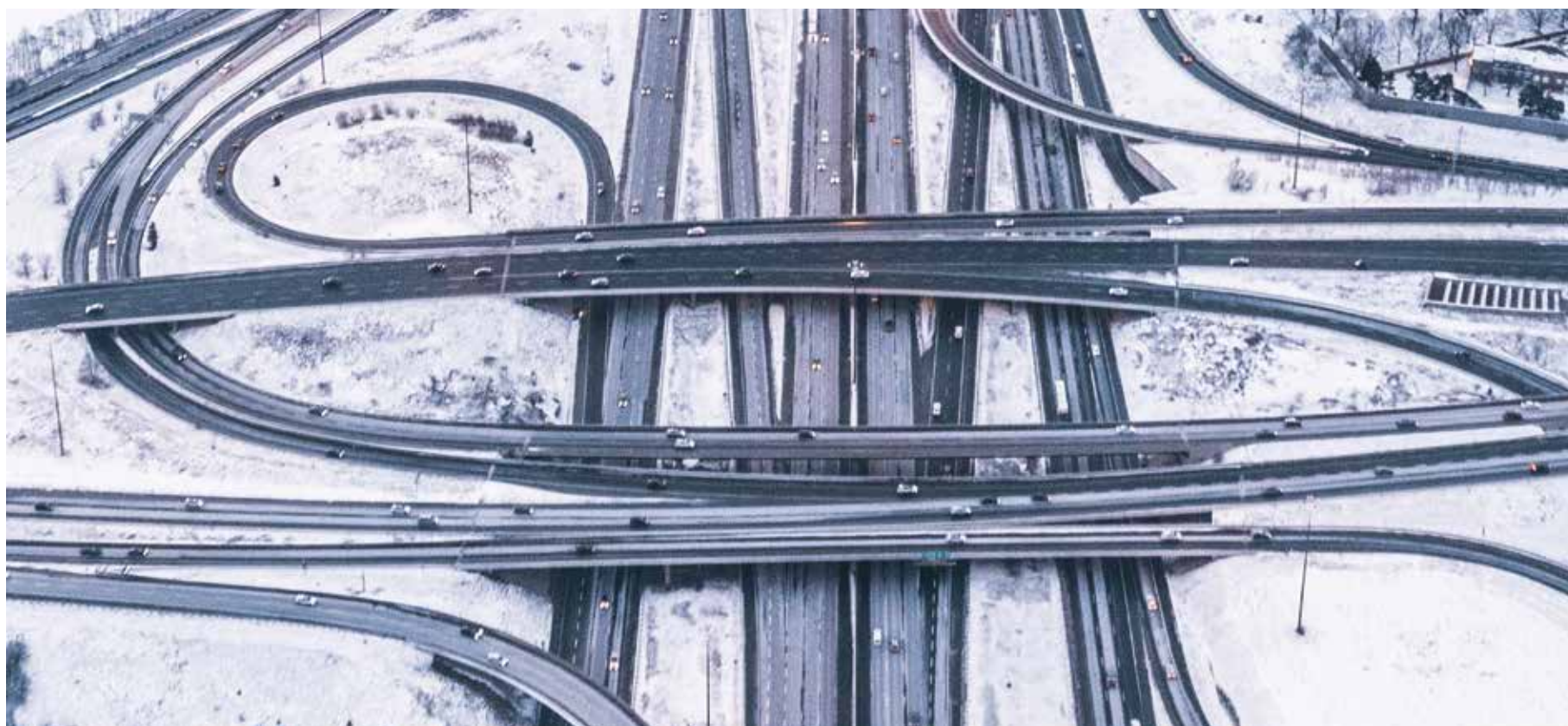
A winter aerial view of Toronto highways. The World Economic Forum's Competitiveness Index shows an alarming decline in Canada's transport infrastructure—our ranking fell from its peak of 10 th in the world in 2008, down to 32 nd in 2019, writes Pascal Chan. Image courtesy of Pexels/Avijit Singh
