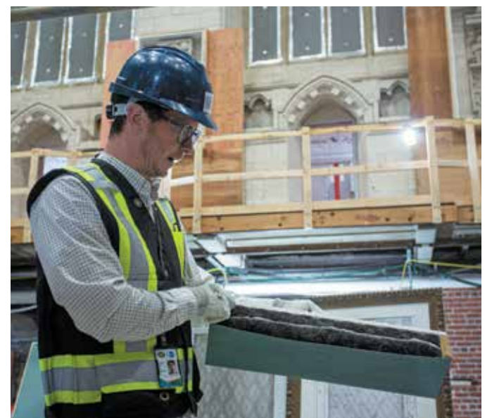
John Legris holds up a cross-section showing the different layers of the House Chamber's painted canvas ceiling. The Hill Times photograph by Andrew Meade
