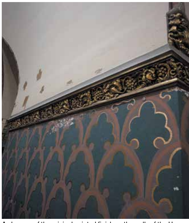
A close-up of the original painted finish on the walls of the House Speaker's dining room. Above are some of the stencil motifs that have been uncovered. The Hill Times photograph by Andrew Meade
