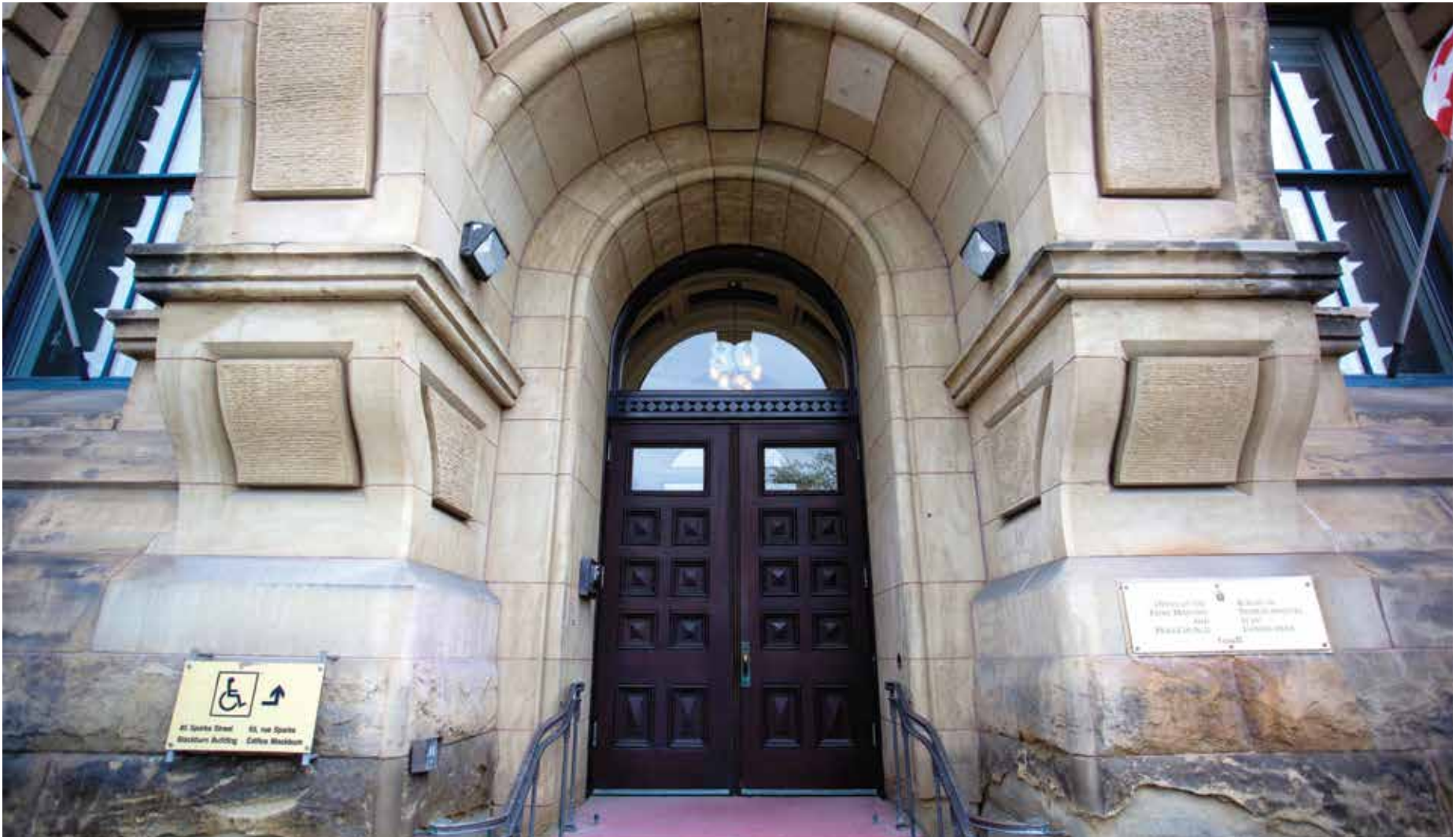
The Prime Minister's Office on Wellington Street in Ottawa. Top public servants will need to show quickly and concretely that they understand the new context, and can steer departments and agencies in a nimble and responsive manner. If they can't, they may find others waiting in the wings to do so in their place. The Hill Times photograph by Andrew Meade
