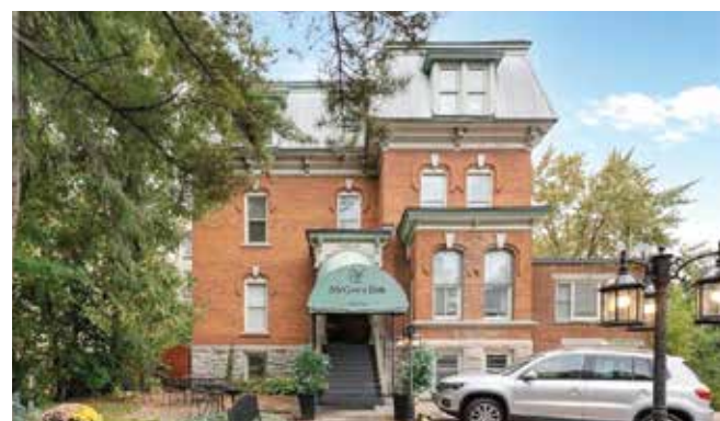
The house at 185 Daly Ave. was built for Canada's longest-serving Privy Council clerk in 1886. Screenshot courtesy of realtor.ca
